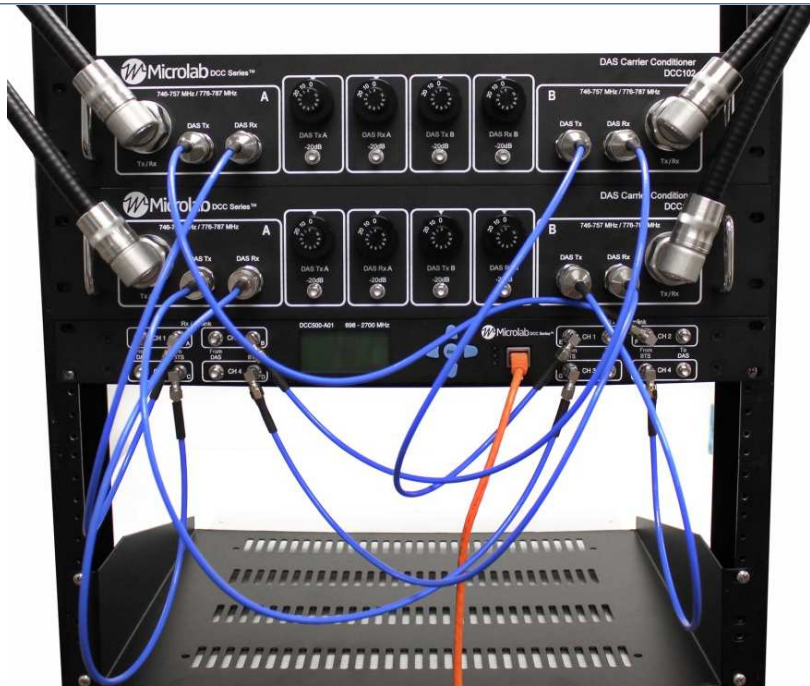
Figure 10 - Example of cabling between legacy DCC102 and DCR
